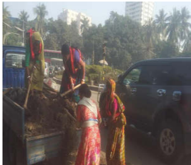
Women working in civil works DMA 616, 14 November,2019
