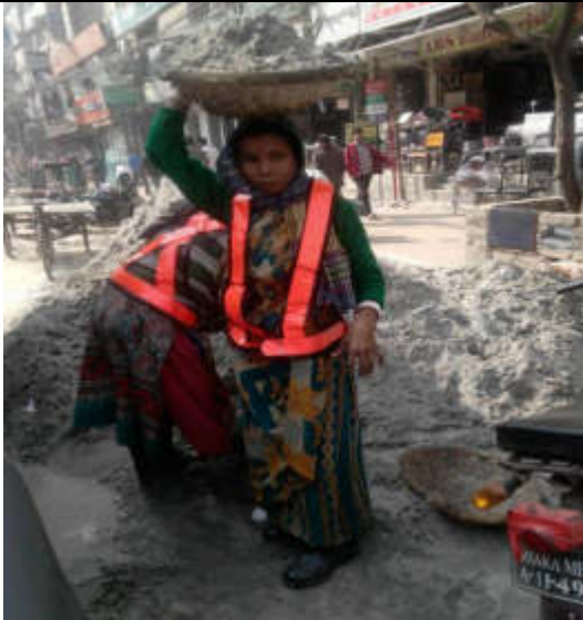
Women working in civil works DMA, 614, October 22,2019
