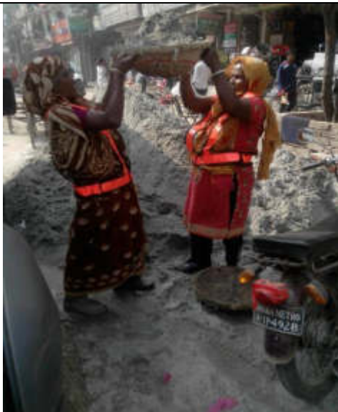
Women working in civil works DMA 615, November 4,2019
