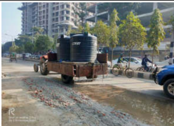
Contractor Pouring water on the road DMA 616, 10 December,2019
